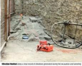
Vibration Meters keep a check on vibrations generated during the excavation and tunneling.
