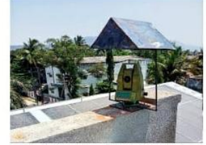
Total Station for measuring settlements and deformations.
