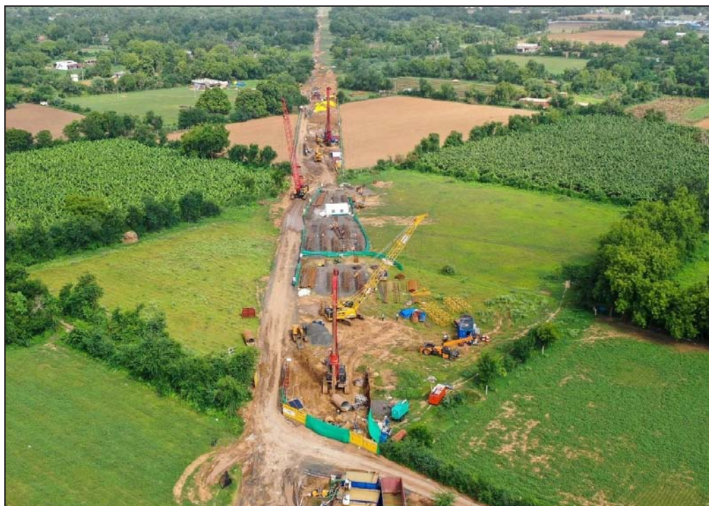
Pile Boring Works at Vadodara, Gujarat.
