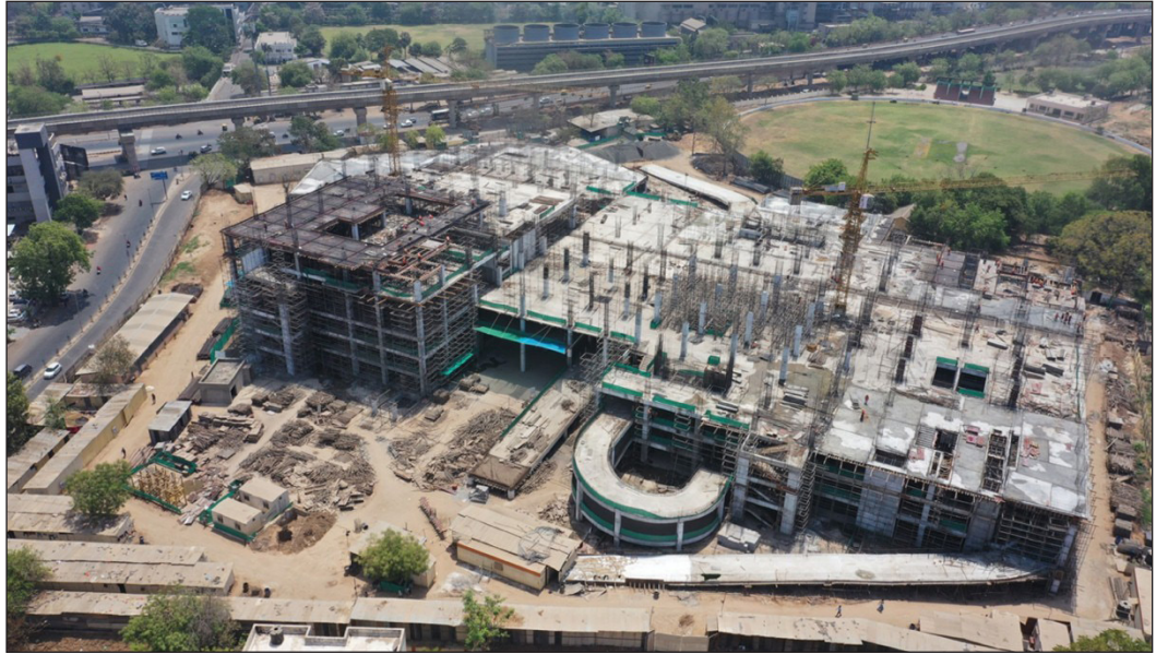
Slab construction at various levels in progress at HSR Sabarmati Terminal, Gujarat.
