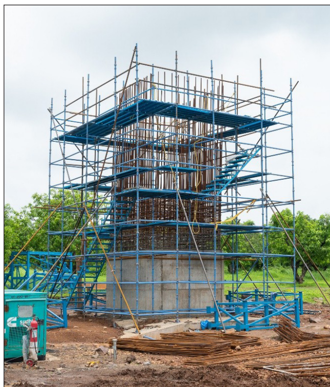
Pier shuttering Work in Progress at Valsad, Gujarat.
