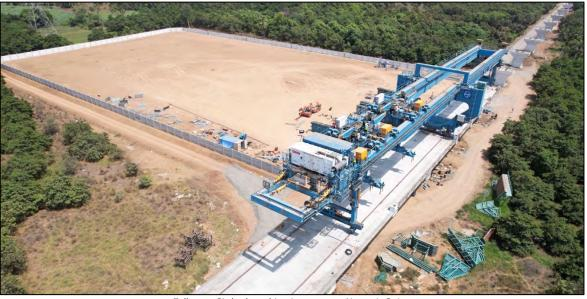
Full span Girder launching in progress, Navsari, Gujarat
