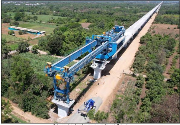
Full span girder launching in progress, Navsari, Gujarat
